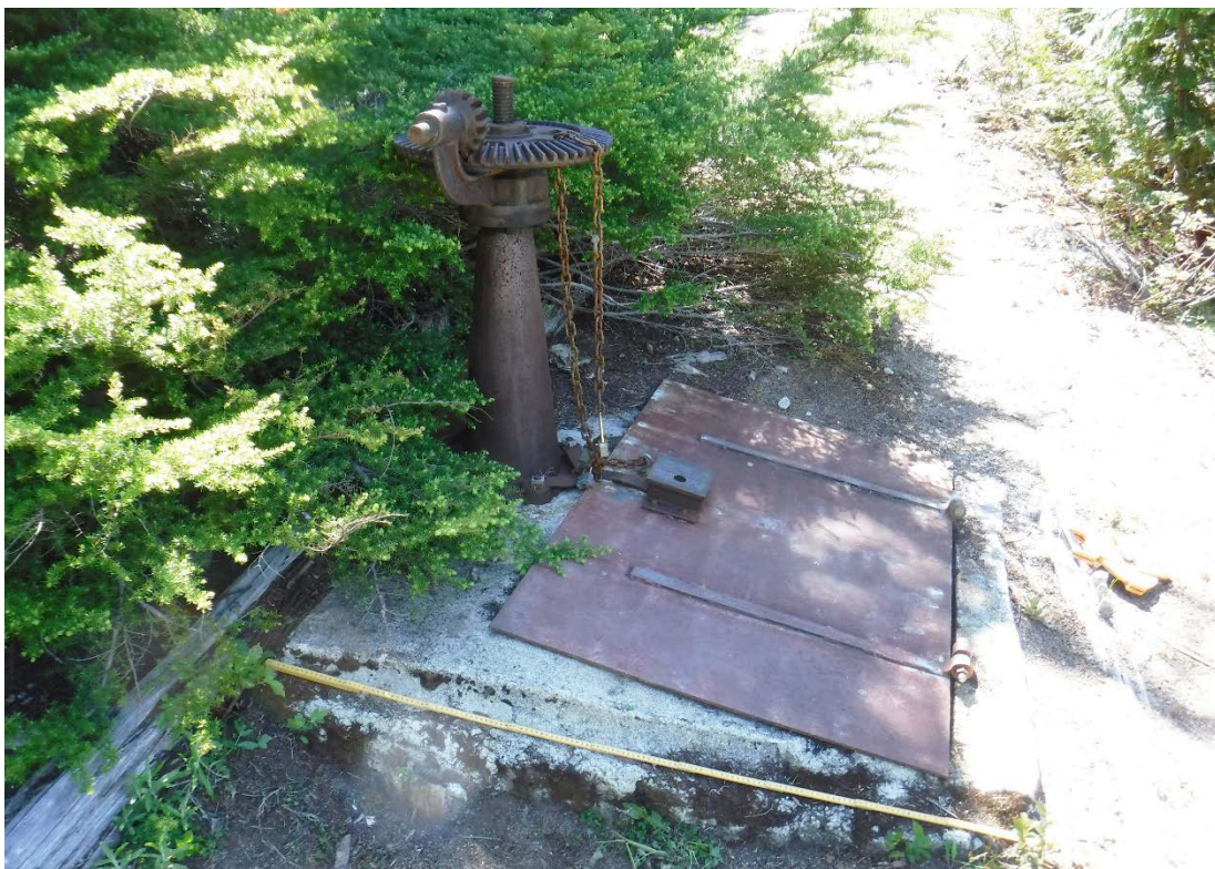
Figure 3-17. Gate Actuator and Gate Chamber near Klonaqu Lake
