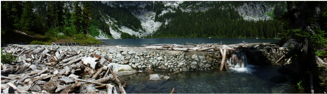
Figure 3-18. Dam Structure at Square Lake
