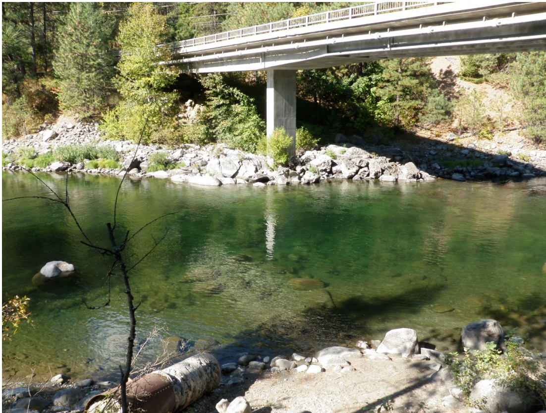
Figure 3-21. Wenatchee River at Icicle Road Bridge near Public River Access
