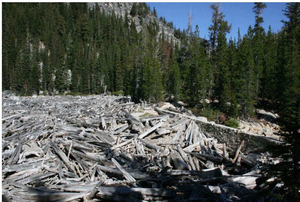
Photo 3. Masonry Dam between Upper and Lower Snow Lake
