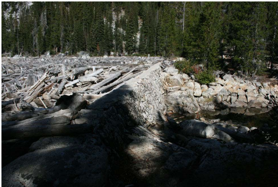
Photo 2. Masonry Dam between Upper Snow Lake (on left) and Lower Snow Lake (on right)
