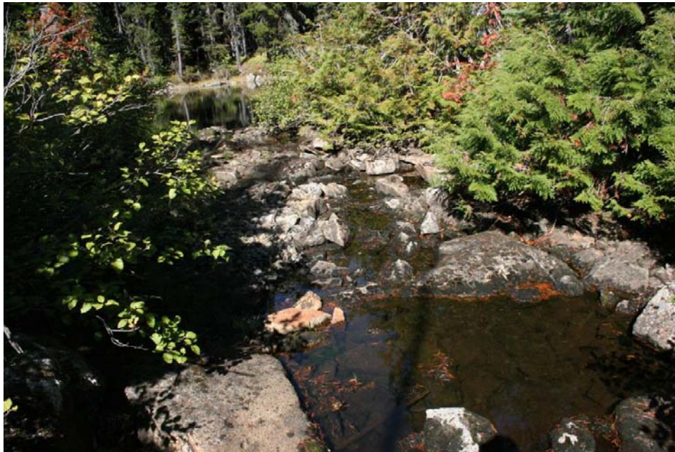
Photo 5. Channel below Lower Snow Lake Dam
