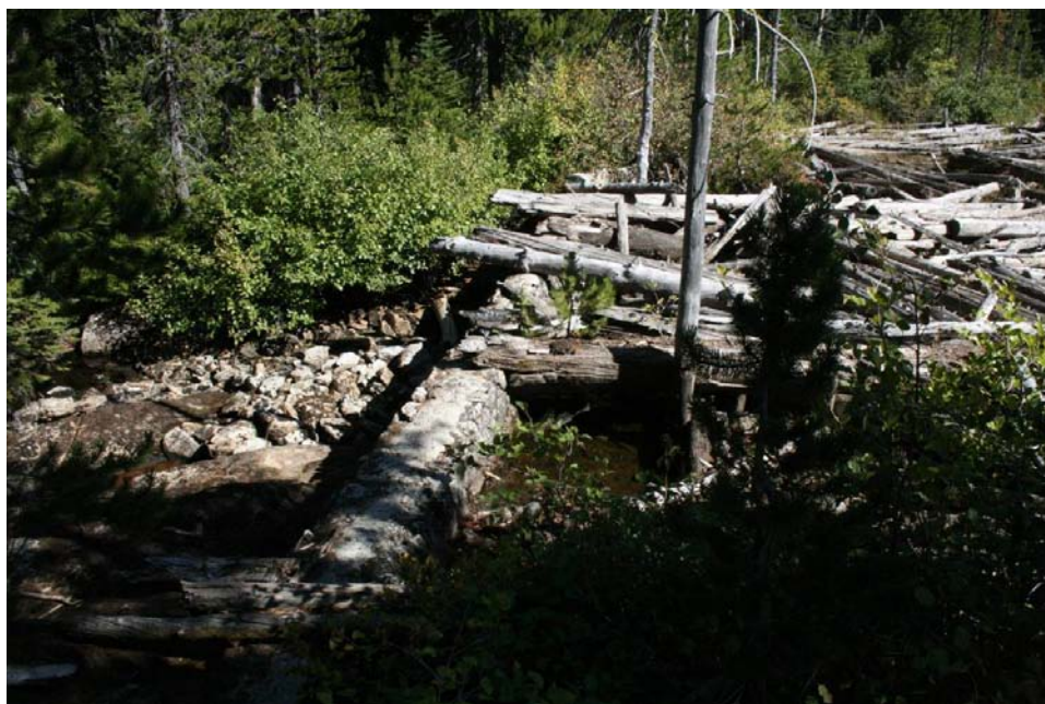
Photo 4. Masonry Dam at North End of Lower Snow Lake
