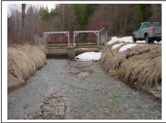
MVID West Old Screen Typical of East Screen
