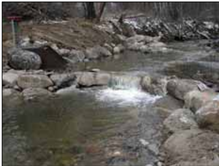
Marracci Weir After
