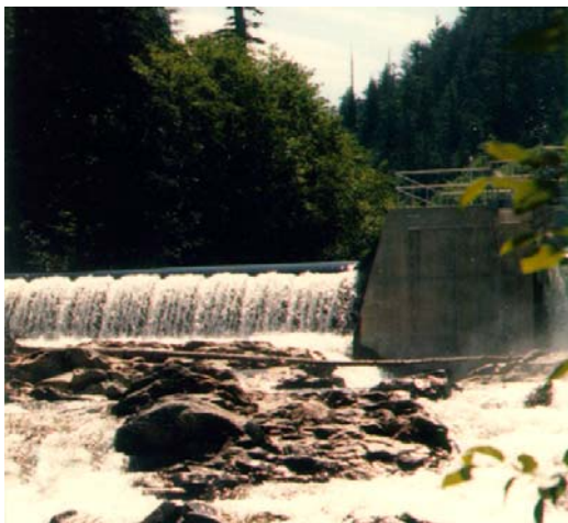
Photograph 3.5-5. Week Falls rubber dam; inflated with water over crest.
