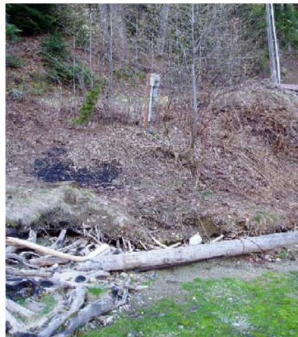
Photograph 5.1-1. Shows septic tank that is located very close to the shoreline and could be impacted by any of the five alternatives.
