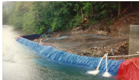
Photograph 3.5-8. Portadam at MWH Wynoochee Hydro Project on the Wynoochee River near Montesano, WA
