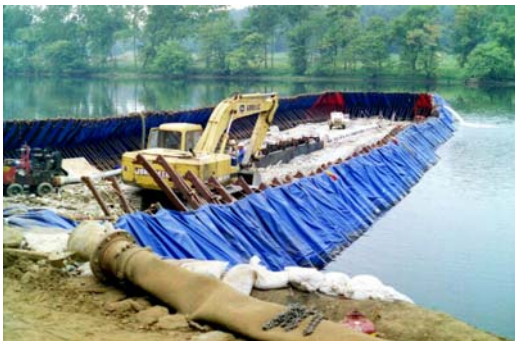
Photograph 3.5-7 Typical Portadam river crossing. (Photo courtesy Portadam, Inc.)
