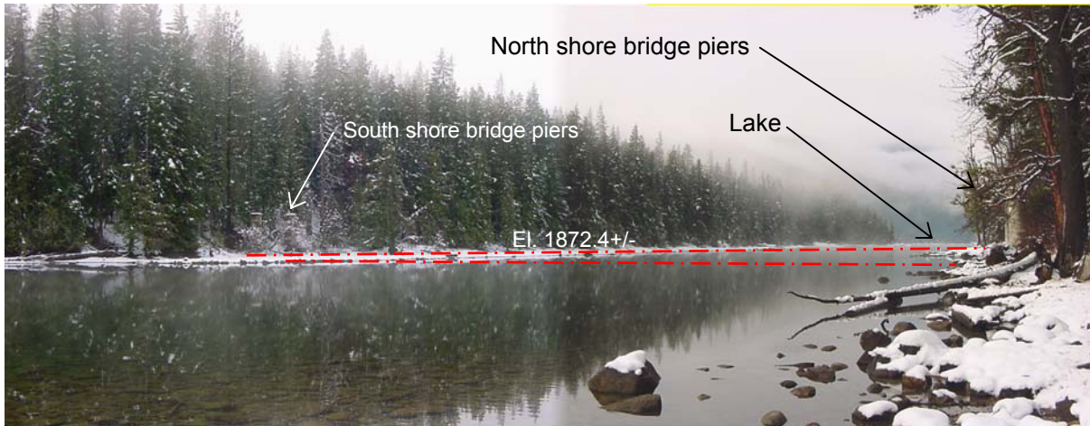
Photograph 3.5-2. Potential location of impoundment structure on Wenatchee River, looking upstream.
