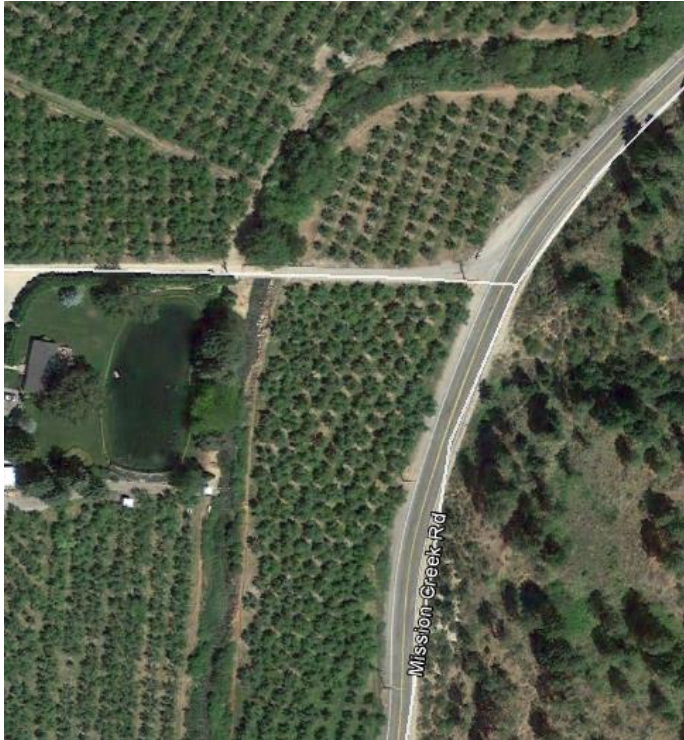
Figure 3. Mission Creek. Google Earth image from 2017 showing bridge where Figure 1 and 2 photos were taken.
