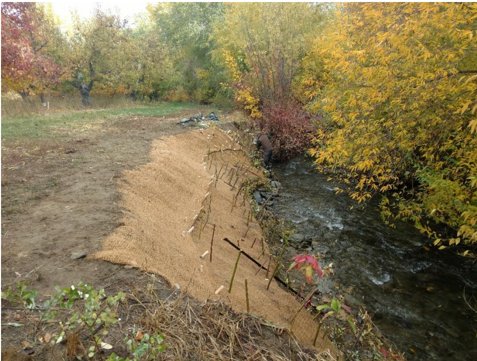
Figure 9. Mission Creek After bioengineering bank stabilization project in 2017. Slope was contoured, coir fabric was tucked under at toe of slope and secured with stakes and soil, willow wattle constructed at toe of slope and live stakes placed throughout the structure.
