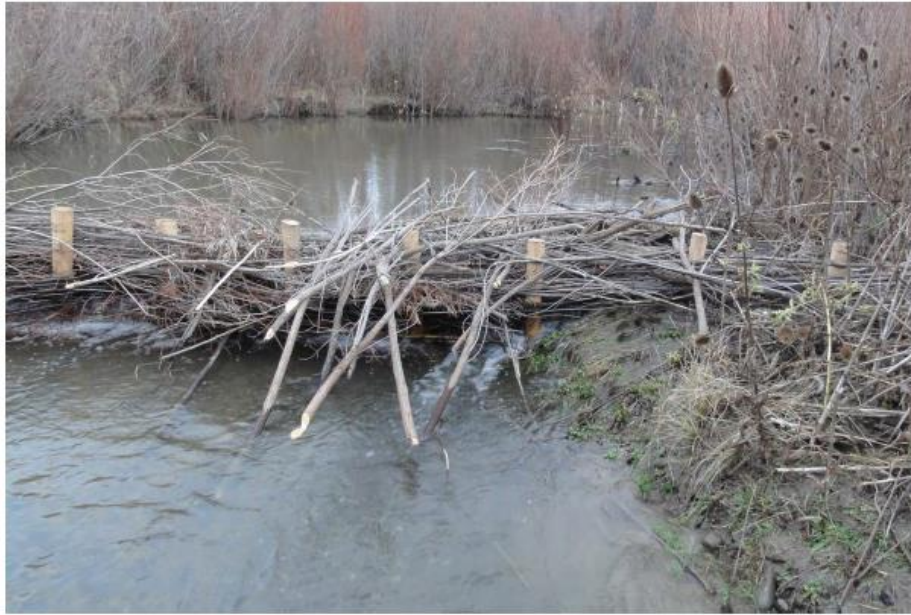
Figure 20. Example of beaver dam analog using a post line and weaving (Photograph from Pollock et al. (2012)).
