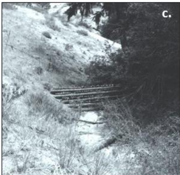
Figure 2. Historical photos from the mid-1900s (a, b, c), compared to photo taken at nearby location in August 2016 (d): US Forest Service sign explaining soil erosion issues and rehabilitation efforts of the 1930s-1950s (a), rock-terrace structure intended to slow hillslope erosion (b), wooden check dam structure intended to store sediment in ephemeral channel (c), inferred location of wooden check dam structures in Peavine Canyon, which are presumed to be complete buried where there are regularly spaced topographic steps along the channel (d).
