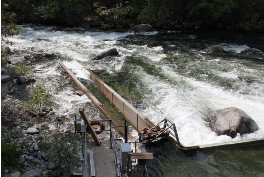
Figure 25. LNFH diversion, fish ladder, and streamflow conditions on July 20, 2012 at a streamflow of 1,271 cfs.
