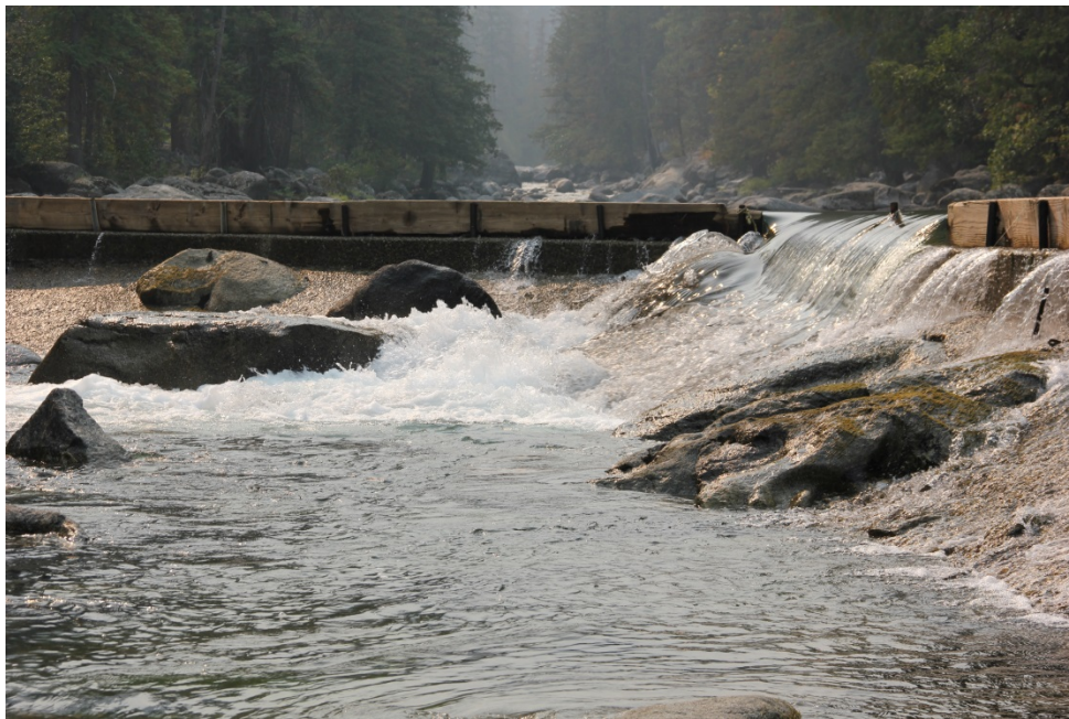
Figure 32. Spill over the LNFH diversion dam in September 2012 at a streamflow of 121 cfs. The notch in the dam flashboards is visible near the right side of the photo.
