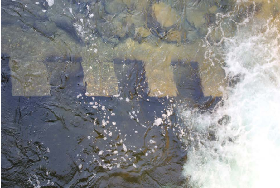
Figure 11. Dentates at the downstream end of the pool below the weir at S2.
