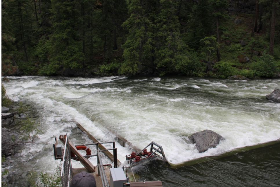
Figure 23. Figure 20.7. LNFH diversion, fish ladder, and streamflow conditions on June 5, 2012 at a streamflow of 2,663 cfs.
