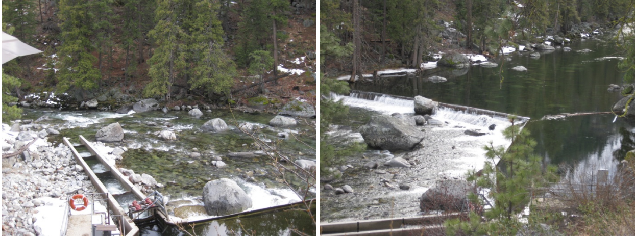
Figure 3. LNFH intake structure located on Icicle Creek at RM 4.5. Left image is looking downstream at the fish ladder and the right image is of the low head dam with the ladder visible in the lower left. The location of the water conveyance channel is not depicted in the figure but it is located to the right and just downstream of the ladder when looking upstream.
