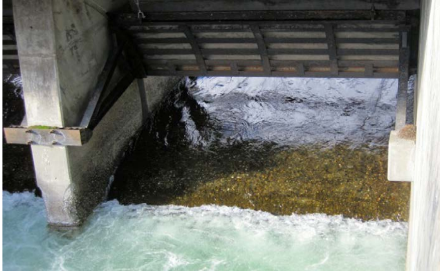
Figure 4. LNFH Structure 2 located on Icicle Creek at RM 3.8. Image is looking upstream at one of two spill bays with the spill gate open.
