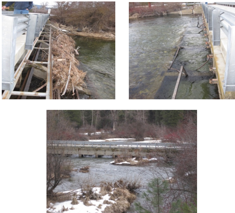
Figure 5. LNFH Structure 5 located on Icicle Creek at RM 2.9. Top left image shows the upstream side of Structure 5 with debris accumulation, top right image shows downstream side of Structure 5 with staff gage on far concrete wall, and bottom image is looking upstream at Structure 5.
