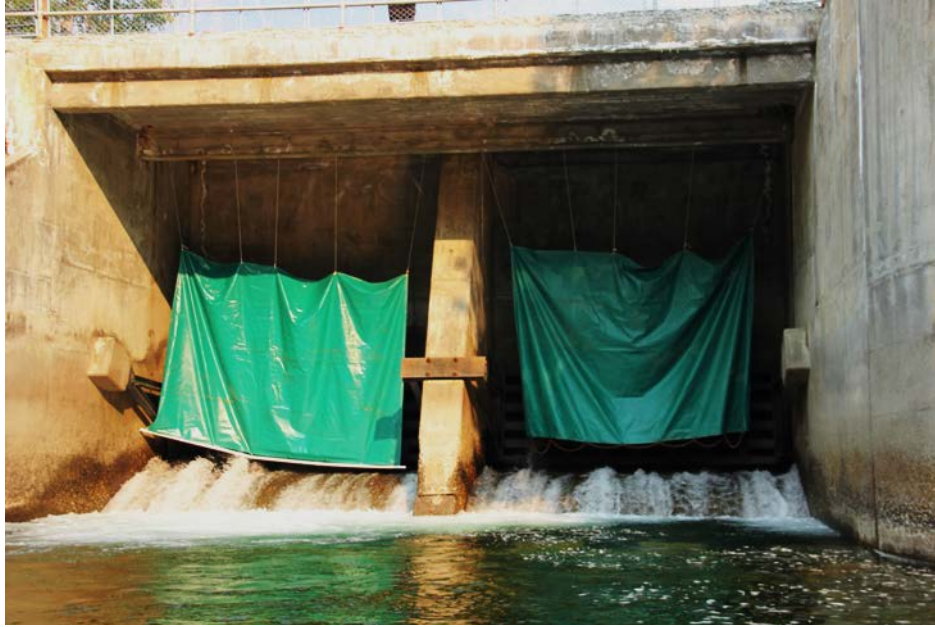
Figure 14. Tarps deployed to protect jumping fish from impact injury on the steel radial gates or the concrete weir.
