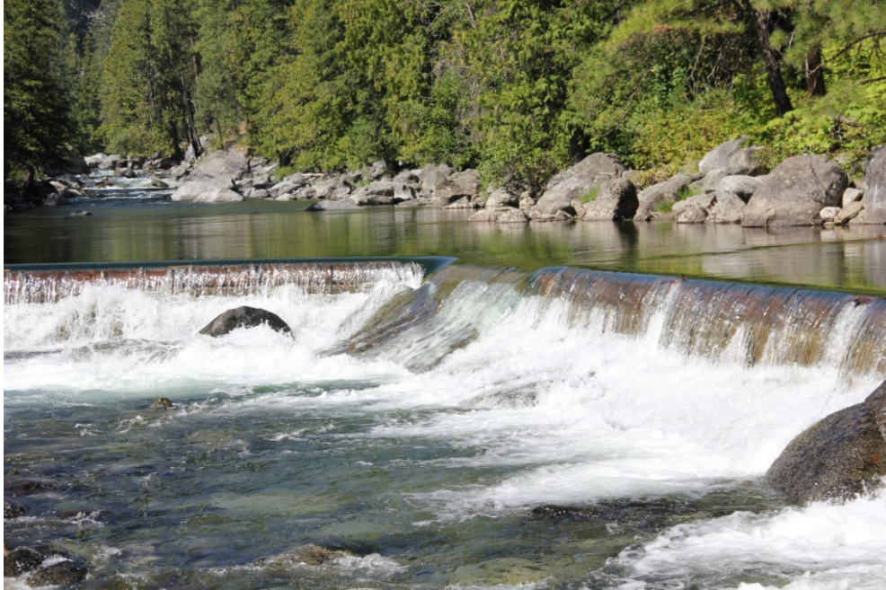
Figure 31. Spill over the LNFH diversion dam in August 2012 at a streamflow of 324 cfs. The notch in the dam flashboards is visible in the center of the photo.
