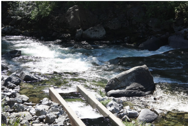
Figure 27. LNFH diversion, fish ladder, and streamflow conditions on August 14, 2012 at a streamflow of 324 cfs.
