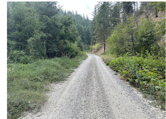
View Road to West
