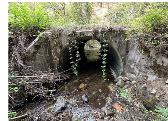
View U/S End Culvert
