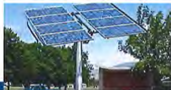
Pioneer Middle School Solar Panels
