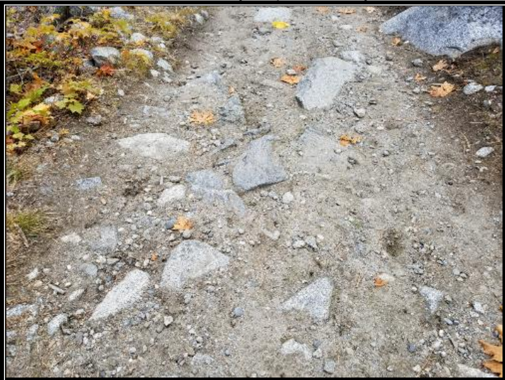
Photograph : view of the existing trail tread showing exposed rock and granular sediments
