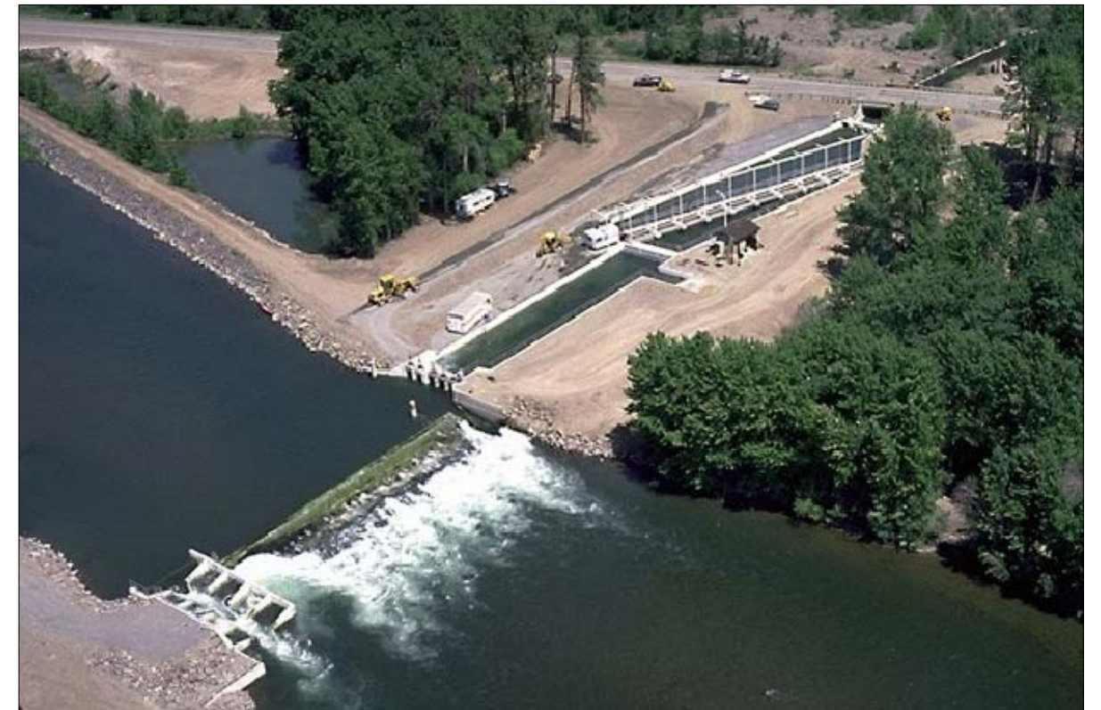
Example of Pool and Chute Fishway on Yakima River
