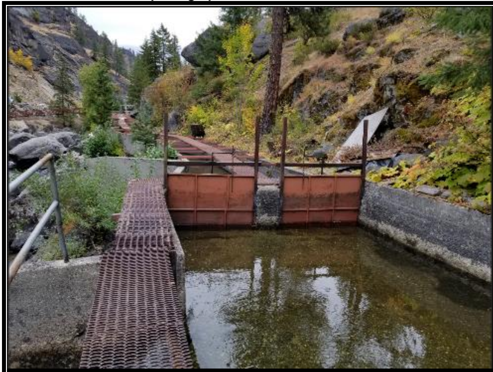
Photograph : Perspective of water control feature south of fish screens. This is north east concrete irrigation district foot bridge to access fish screens from the access road on the opposite side of the creek. This is visible in rear of photograph
