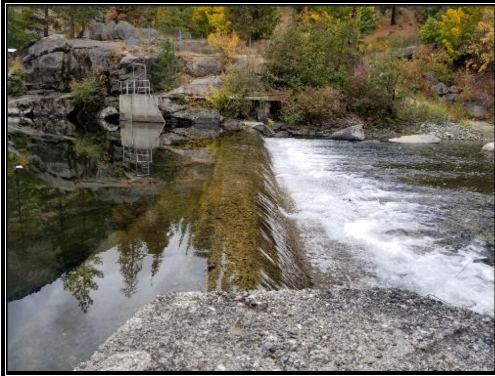
Photograph : view of west bank of creek at diversion dam and vicinity of earthen intake structure. Photograph taken from opposite side of creek looking east.
