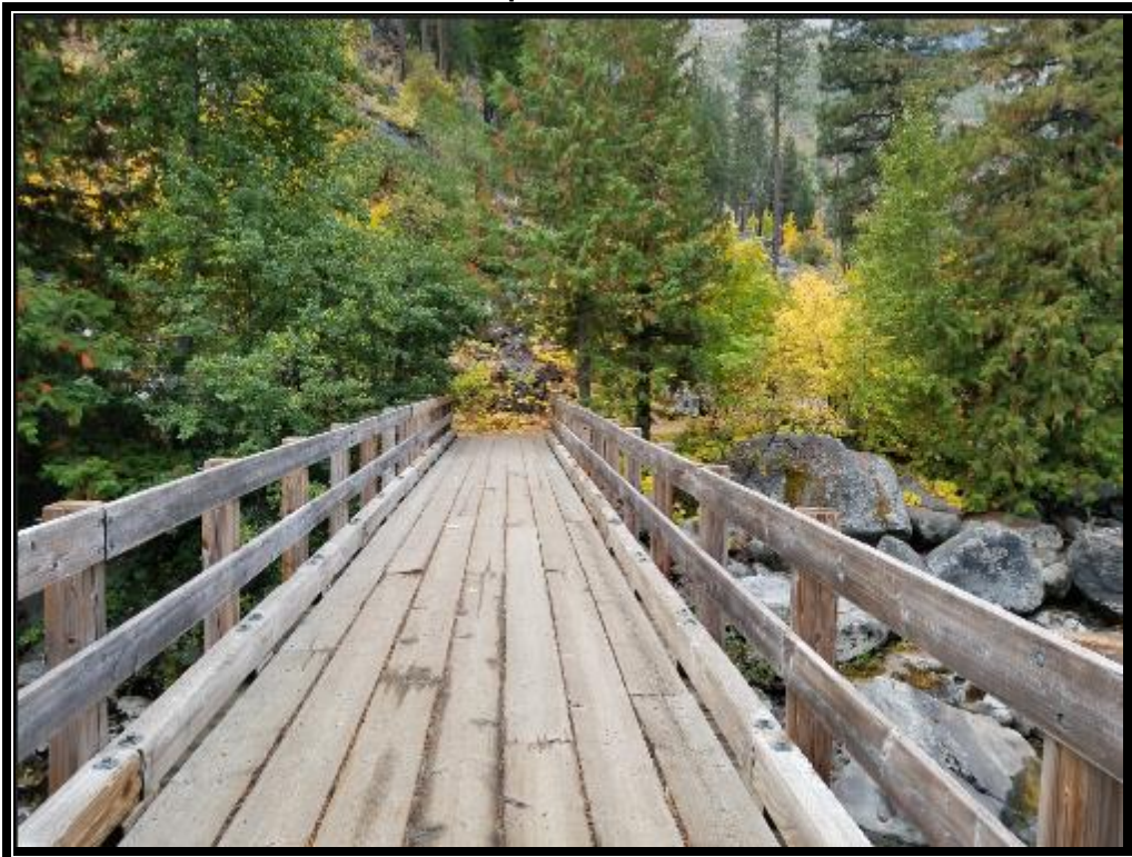
Photograph : view of the Snow Creek foot bridge along the east boundary of the project area. The approaches to the bridge may need some widening. Work could take place in the previously disturbed approach areas at either end of the bridge. View is north.
