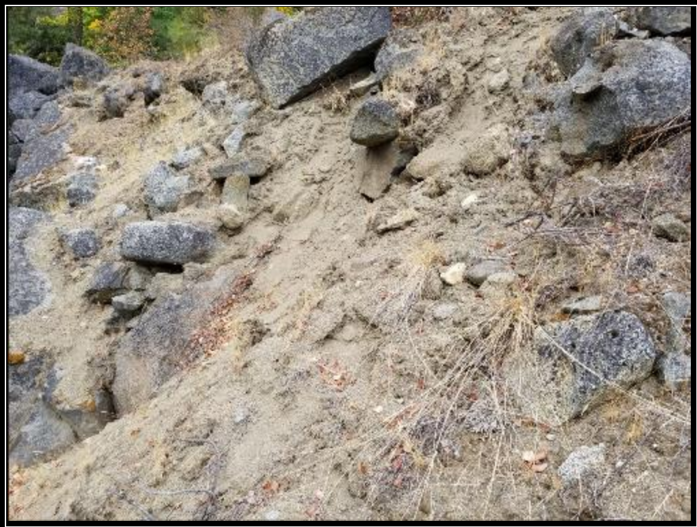
Photograph : Erosion of steep bank observed along north side of creek in fish passage project.
