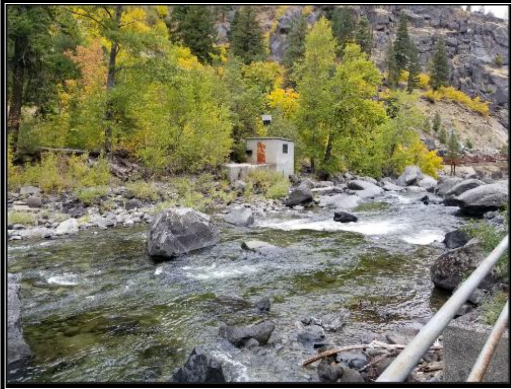
Photograph : Aerial view of location of Screen House and surrounding river bank taken from spiralay on cic e rrigation ana lise is north
