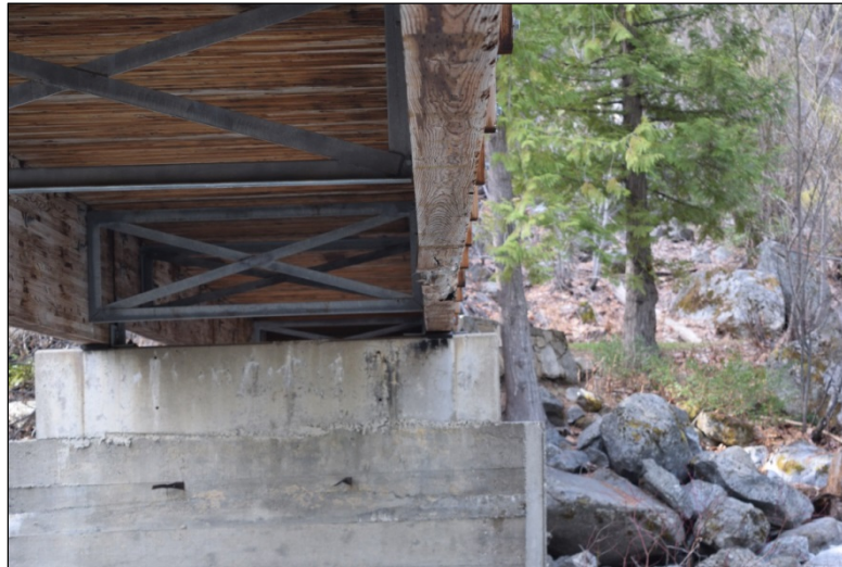
Photo 4: Damage to Existing Stringers Due to Flood Debris
