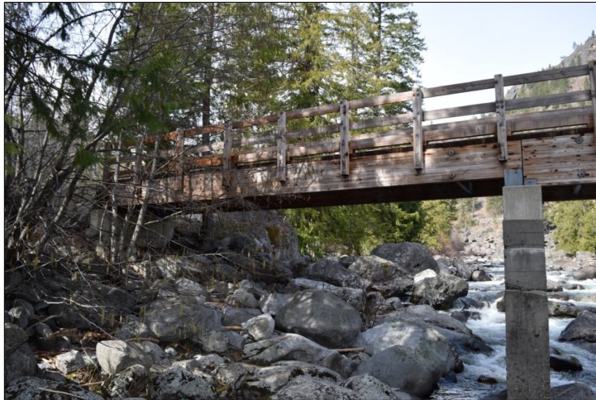
Photo 2: Existing Structure Forest-Side End Span
