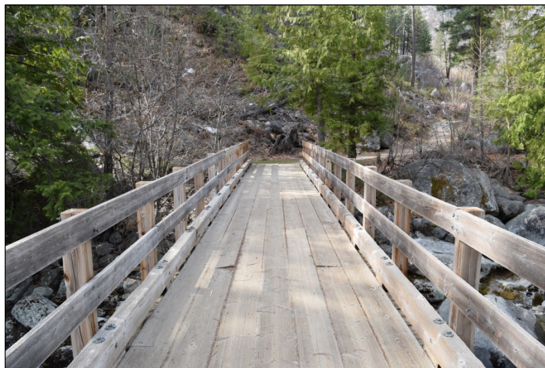
Photo 5: Existing Deck System
