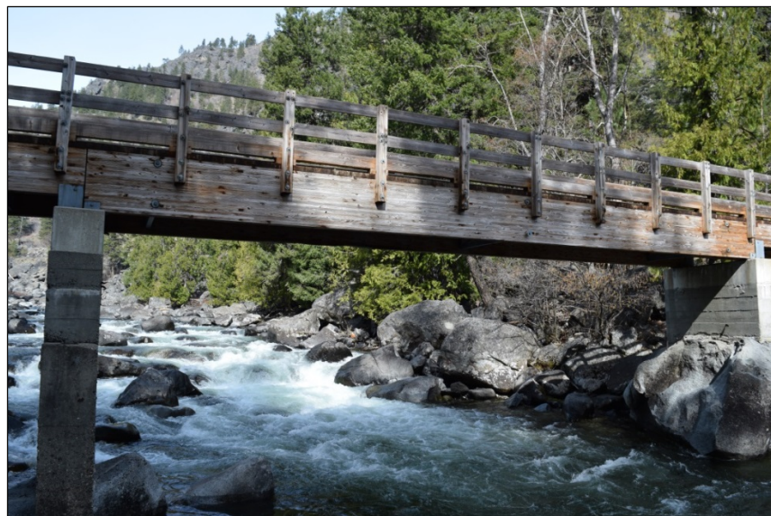
Photo 3: Existing Structure Center Span
