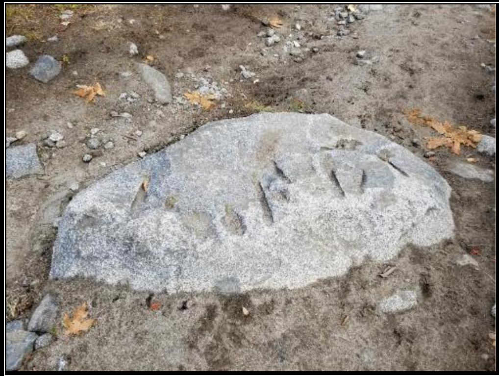
Photograph : partially exposed boulder in the trail tread that has blasting scars on the exposed surface
