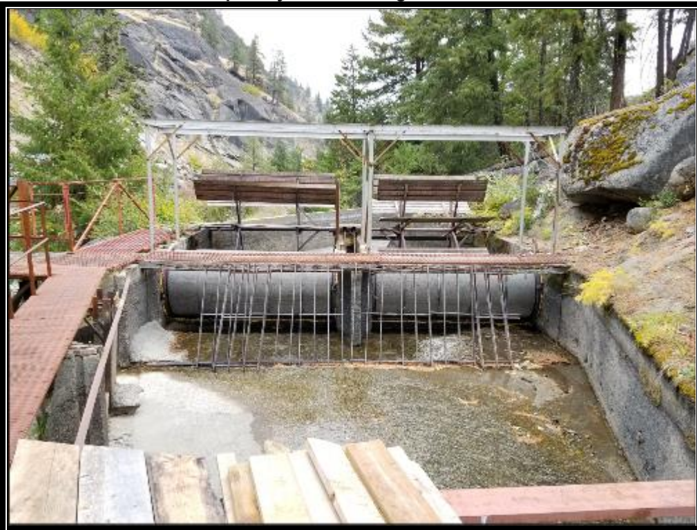
Photograph : Aerial view of existing fish screens located approximately 100 feet north east of cic e creek diversion
